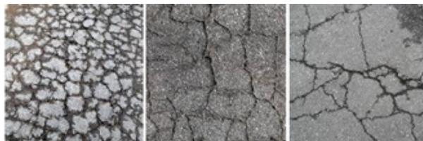
Figure 2: Examples of block crack defect.
