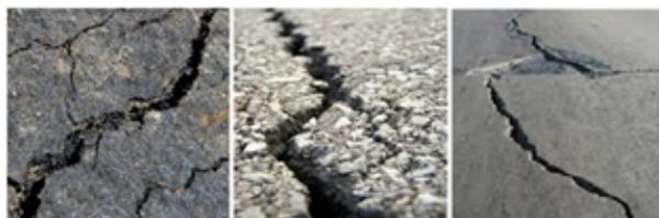
Figure 3: Examples of longitudinal defect.
