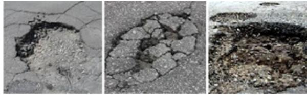
Figure 4: Example of potholes defect.
